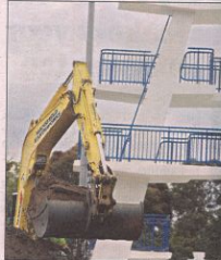
Heavy machinery near the dive pool.
